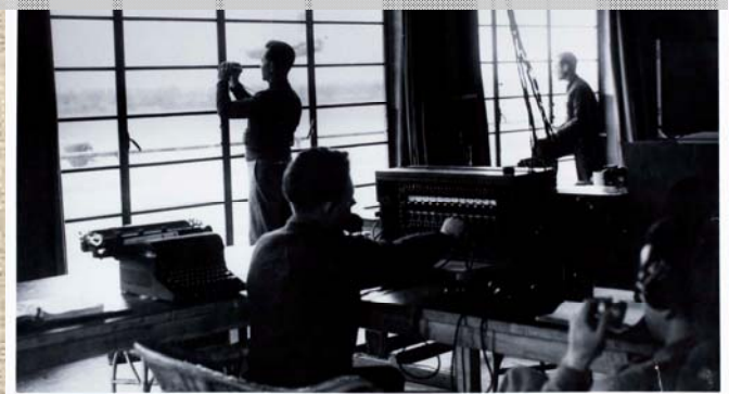
Photograph of a Control Tower. NRO, MC 371/7
